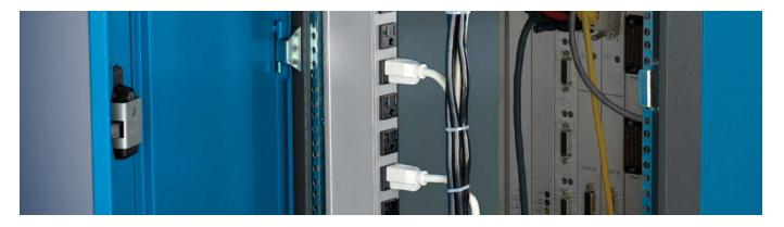
Power Commander® Series High Amperage Units (PDUs) have multiple circuits to provide increased capacity for today's high density server racks. Embedded or remote ammeters are available to monitor current draw.
