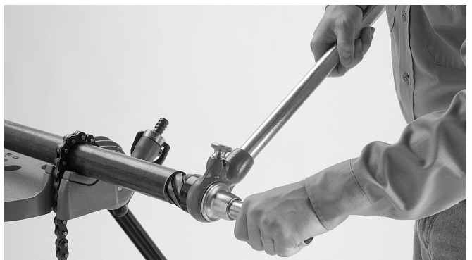
Figure 4 – Reaming End Of Pipe
