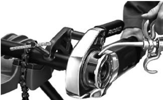
Figure 6 – Threading Pipe and Applying Oil
