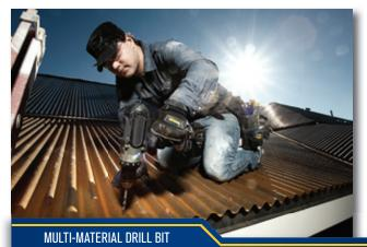
IRWIN Multi-Material drill bits drill through just about any type of material out there – brick, block, tile, metal, wood, plastic and marble. They'll even drill through multiple materials at the same time. These versatile bits are designed specifically for rotary drilling, but are tough enough to be used with hammer drills.
