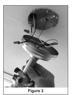
**3.** Securely connect the bare copper (Ground) wire to the (hex-head) screw located on the Crossbar. Securely connect the white lamp wire to the white supply (neutral) wire using wire nut supplied. Securely connect the black lamp wire wire to the black supply (hot) wire using wire nut supplied. (Figure 3)
