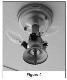
**4.** After connections have been made, carefully push leads into the outlet box. Carefully fasten the Fixture over the Threaded Rods with the Lockwashers and Knurled Nuts provided. Install light bulbs (not included, 60 watt max each). (Figure 4)
