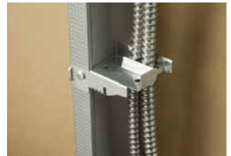
Metal Stud with MC/AC Cable
