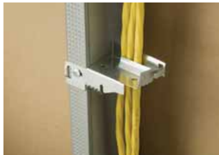
Metal Stud with Non-metallic sheathed cable
