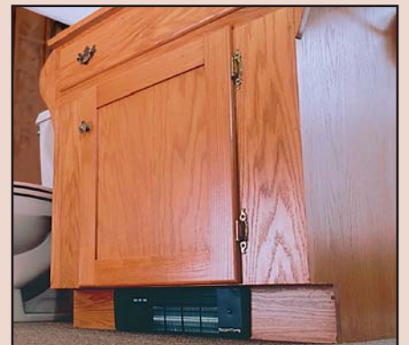
Twin-Flo III heater bathroom cabinet installation.
