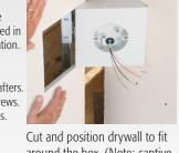
around the box. (Note: captive screws in box.) Install fan or fixture per manufacturer's instructions using captive installation screws.
