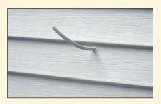
Select location for light fixture and caulk opening around cable.
