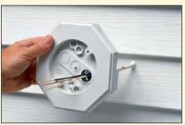
2 Remove knockout from electrical box and insert cable connector. Push cable through connector and position mounting block onto siding.
