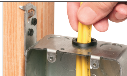
2 Insert cable(s) into individual openings.
